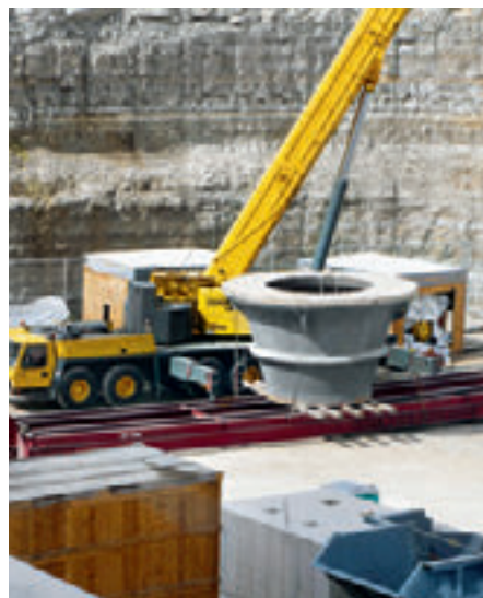
Assembly of the grinding table
