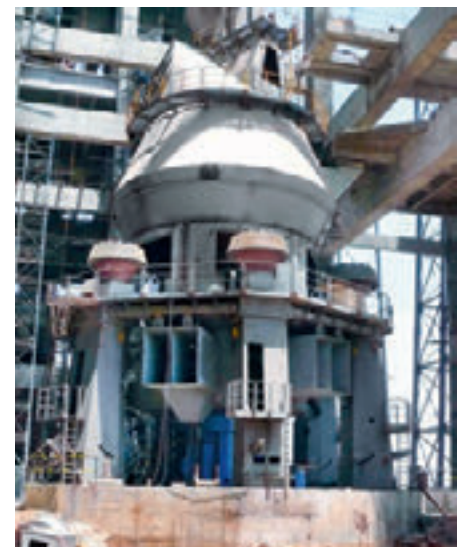
Mill with classifier under construction
