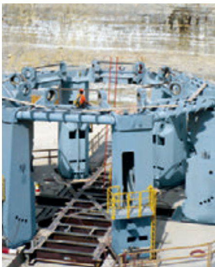
Assembly of the lower part of the mill
